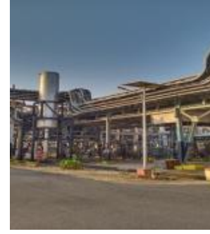
Solar Unit at Plant
