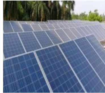
Roof of Central Canteen
