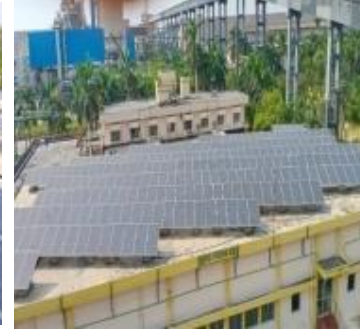
Roof of Control Room
